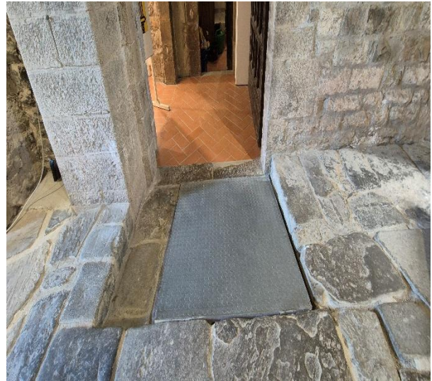
Figure 32 Toilet access ramp
