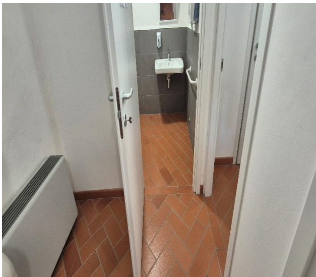
Figure 33 washbasin and door
